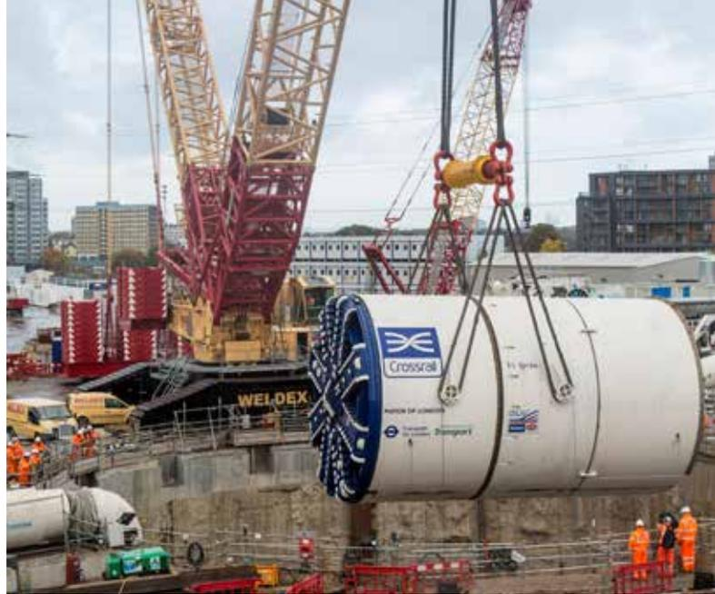
*Lowering a Tunnel Boring Machine into the shaft (Crossrail 1)*
