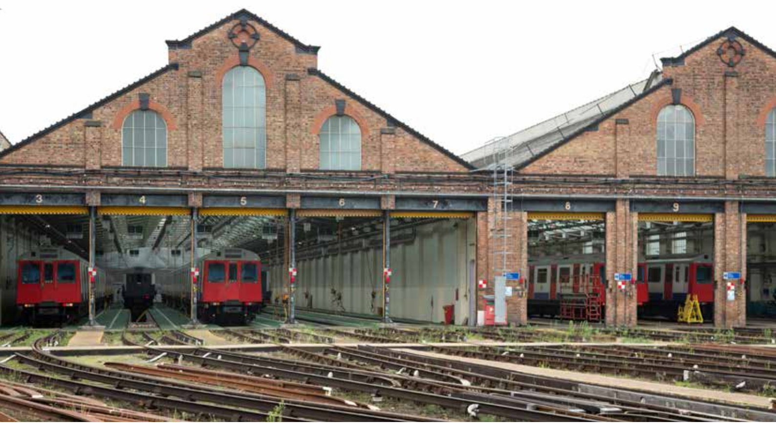
Example of London Underground train depot for District line trains
