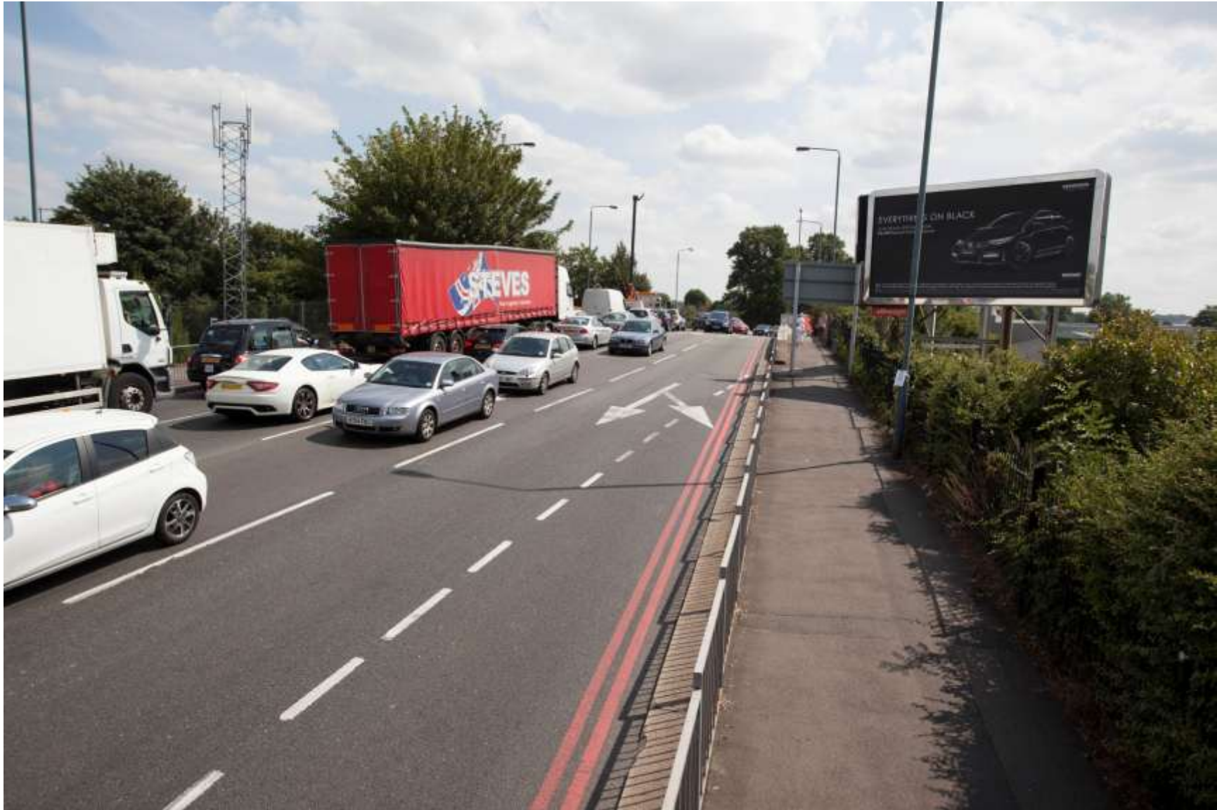
Existing view of A23 bridge
